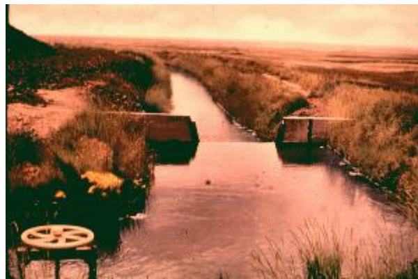
Figure 5-13 -- Cipoletti weir operating with good flow conditions in the approach pool.
