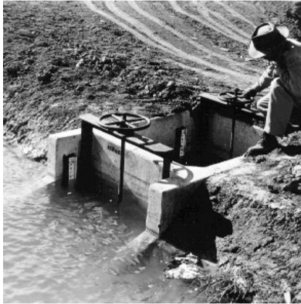
Figure 9-3 -- A single-barrel CHO turnout.
