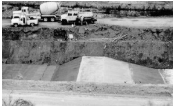
(a) Long-throated flume (broad-crested weir) under construction.
