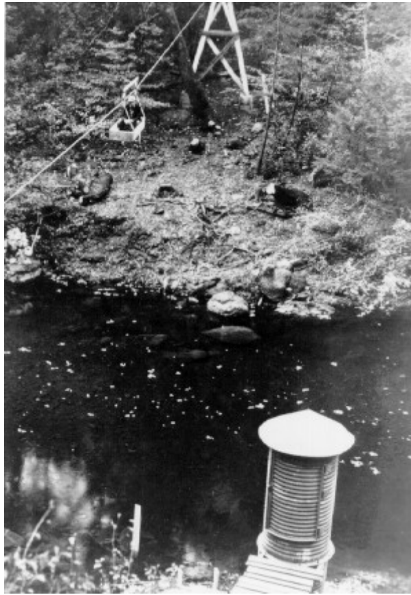
Figure 6-11 -- Current-meter gaging station with cable car, corrugated steel shelter house, and stilling well.
